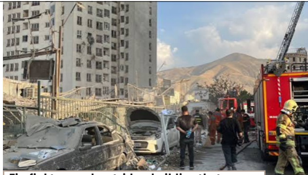
Firefighters work outside a building that was hit by Israeli air strikes north of Tehran
